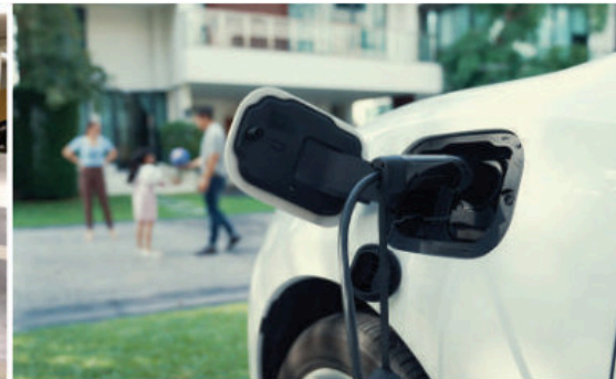
EV charging points in parking
